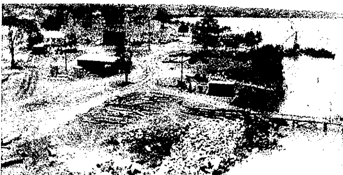
The site of the Port construction process and workers barracks. Photo courtesy of the Strathdee Family.
